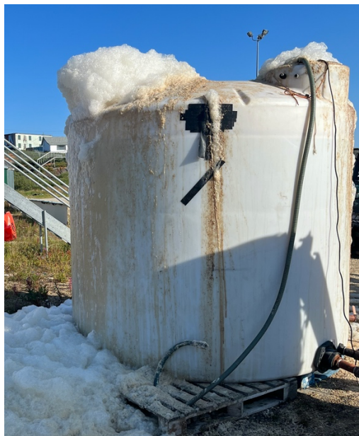
Figure 5.1: Churchill 9000 liter bioreactor, exhibiting high foam production as a result of aeration and bacterial growth, noting the green airline providing air to the venturi system.
