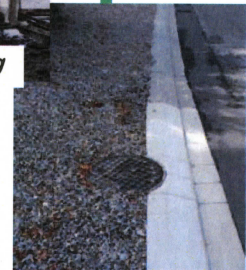
"typical" dewatering well infrastructure
