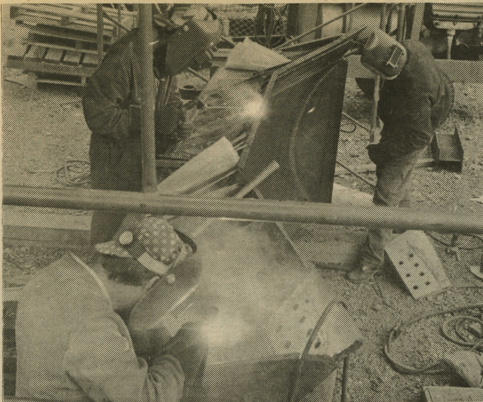
WELDING TRAINEES, working in three-man shifts, are shown as they reconditioned a huge U-shaped blade from a D-9 tractor used in moving crushed rock in an open pit mine. The blade was shipped to Cariboo College from the Rossland Mining School, lifted into the outdoor welding area by means of a 15-ton crane,
