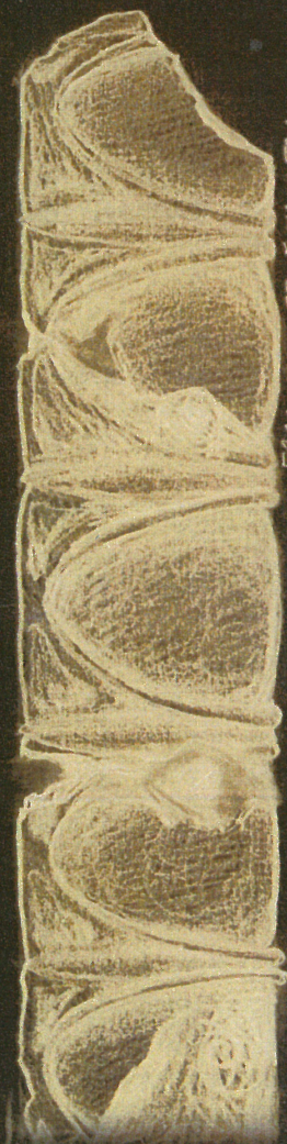
IONIC CORINTHIAN CAPITAL FROM ENGAGED COLUMN (ELEVATION #2) CAST TERRA-COTTA PAINTED WHITE. POSSIBLE SPANISH INFL.
