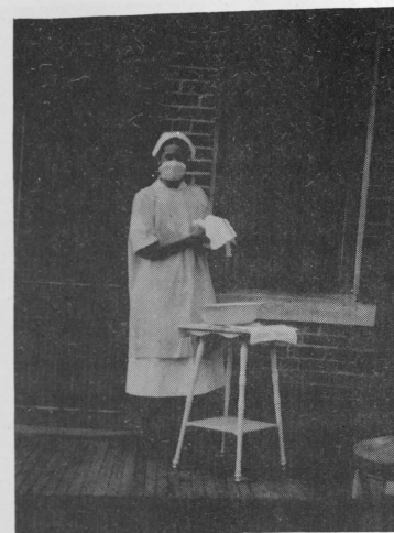
On the steps of Isolation Hosp.
